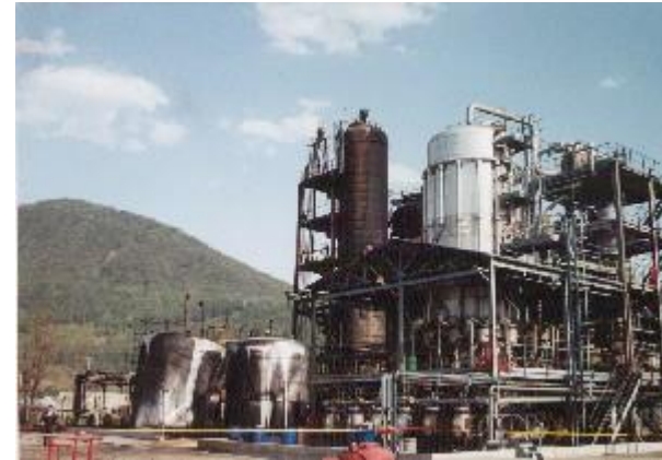
Factory explosion (Jarrie - [Isère] France)
